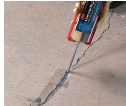
Fix cracks, spalls, and breaks in concrete:
